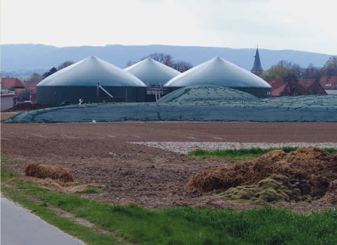
Figure 1: Biogas plant in Adensen near Hildesheim, Germany (Photograph: Lorey)
