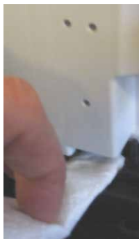
Fig. 40: Drying the leak sensor
