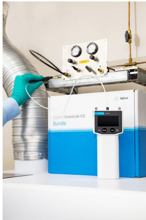
Figure 10. Example of using the Agilent CrossLab CS Electronic Leak Detector to check argon gas fittings.
